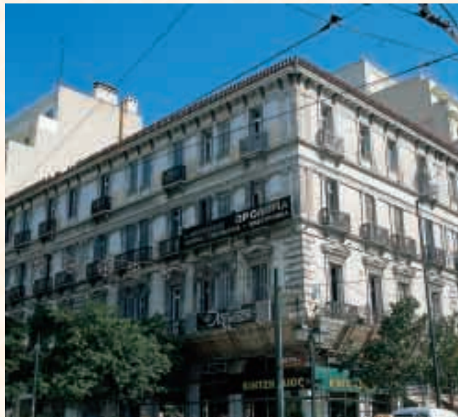
"Hatzikyriakeio". Renovation of an office building (3,600 sq. m.)
