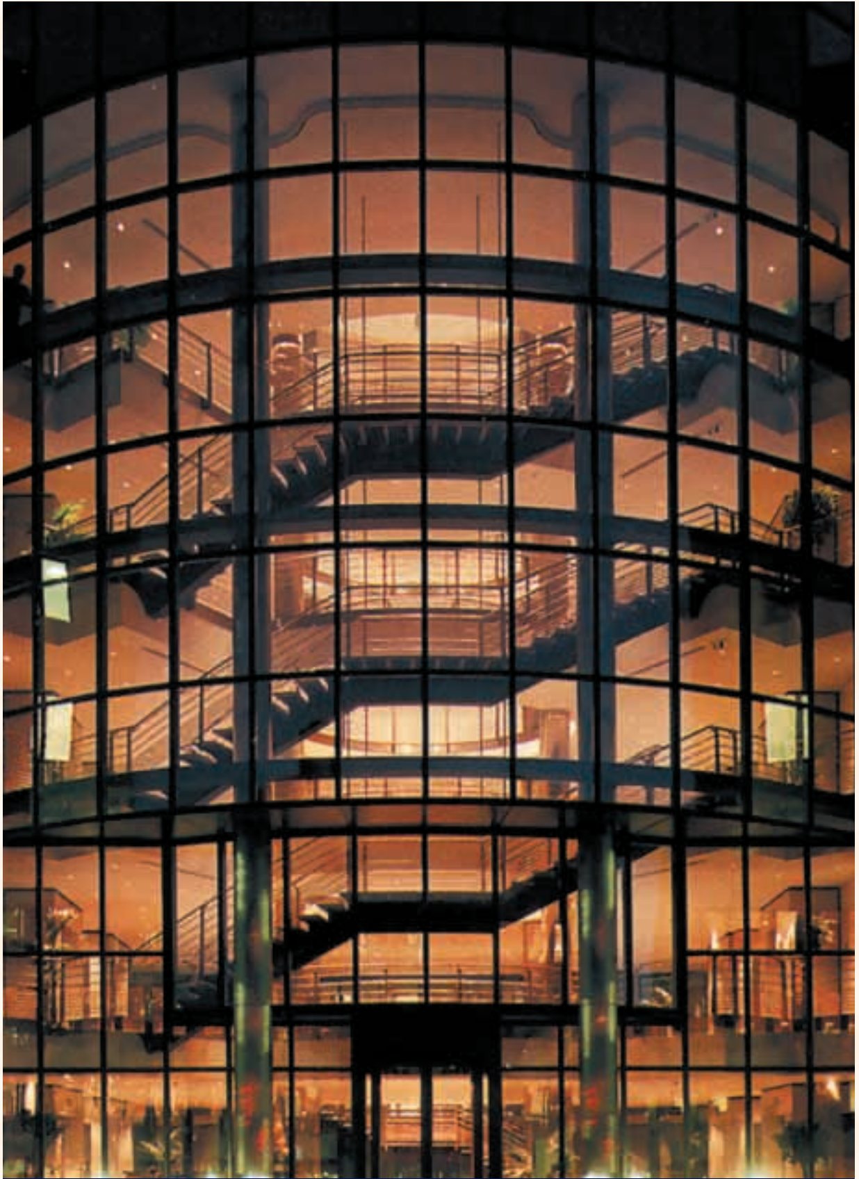
IIK building, with floor space of 17,000 sq. m. in Luxembourg
